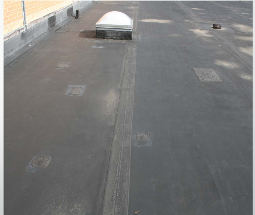
23 year old, aging and patched roofing on MS/HS
