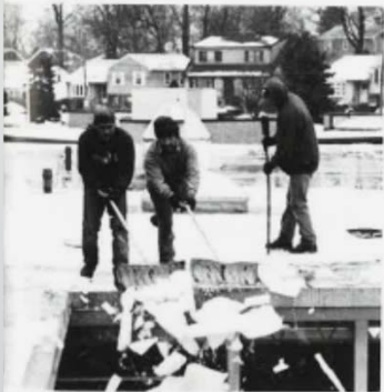
Chopped ice and snow are heaved off the roof to prevent further leaks and damage.
