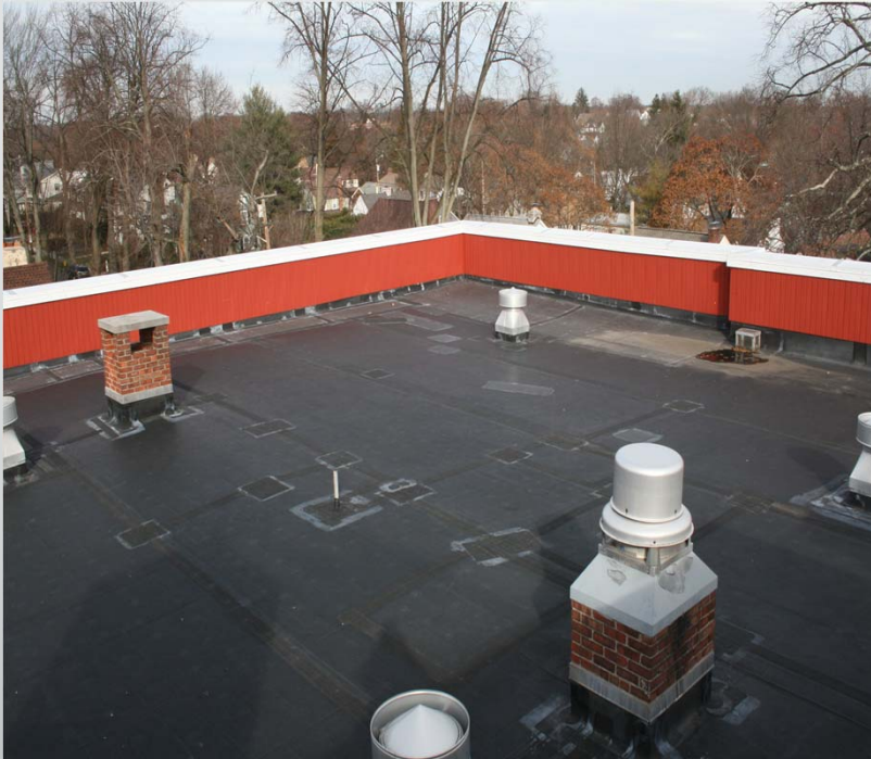
Patched roofing and seams at F.E. Bellows
